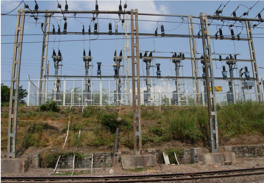
Sectioning and Paralleling Post (SP)
