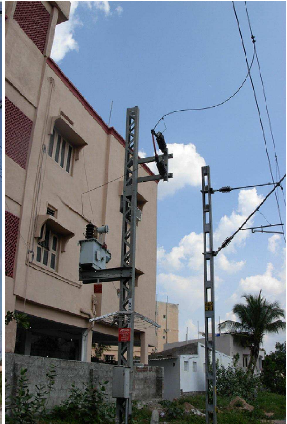
AUXILIARY TRANSFORMER (AT)
